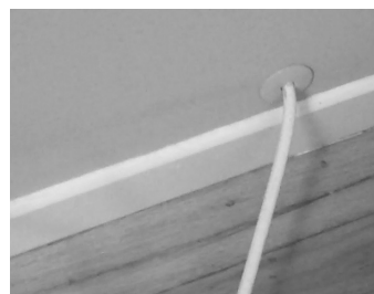
Locate coaxial cable coming into the house. (i.e. from cable or satellite provider).
